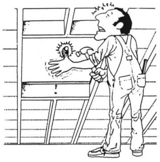
Framing the opening. Check rafter or trusses for dimensions of lumber. Using lumber of the same dimension, frame under deck across opening, to connect rafters or trusses. Form square or rectangle to exact dimensions of opening.
